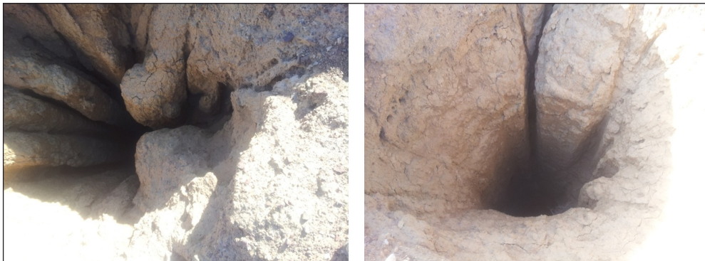
Figure 6 Qanat wells near Khavarshahr with 2 m diameter and about 12 m depth, on the PS2-d scarp. The placement of lake sedimentary layers on high-permeability sediments (Series B) has caused the subsurface water to flow beneath these sediments. The ancient people passed through impenetrable units and built the horizontal channel of the Qanat between these two sedimentary units by digging the qanat to reach the lower layer. Most of these wells and qanats have collapsed and been blocked due to subsurface erosion of tunnels and subsequent qanat collapse. Qanats have now been OSL dated to about 4,000 years BP. They provide a lower limit bracketing date for the lake sediments.
